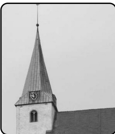
Would you have known? Disguised base station in a spire
